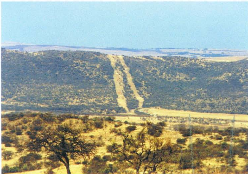
Figure 15: Typical scarring caused by installation of a pipeline
